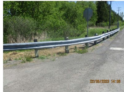
Southwest SBGR - Collision Damage
