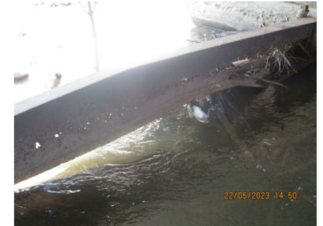
Footing Bracing – Severe Section Loss
