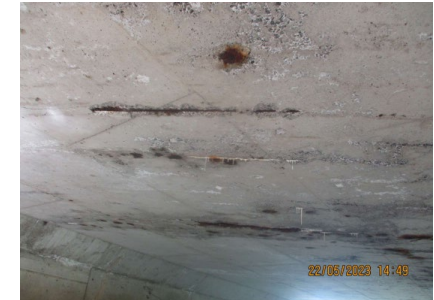
Interior Soffit – Medium Delamination
