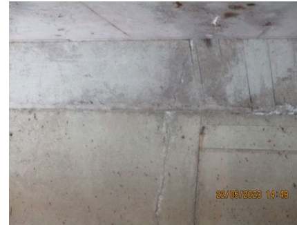
Wide Vertical Crack on South Abutment
