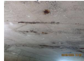
Interior Soffit – Medium Delamination
