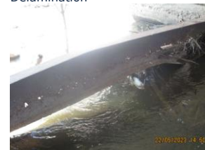
Footing Bracing – Severe Section Loss
