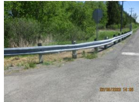
Southwest SBGR - Collision Damage
