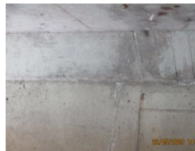
Wide Vertical Crack on South Abutment
